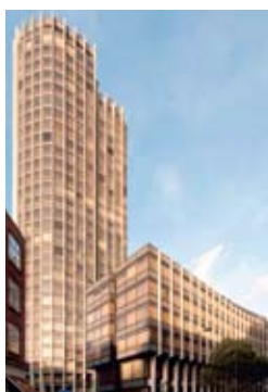
Kings Reach Tower, SE1: CIT and Jadwa purchase for £60m
